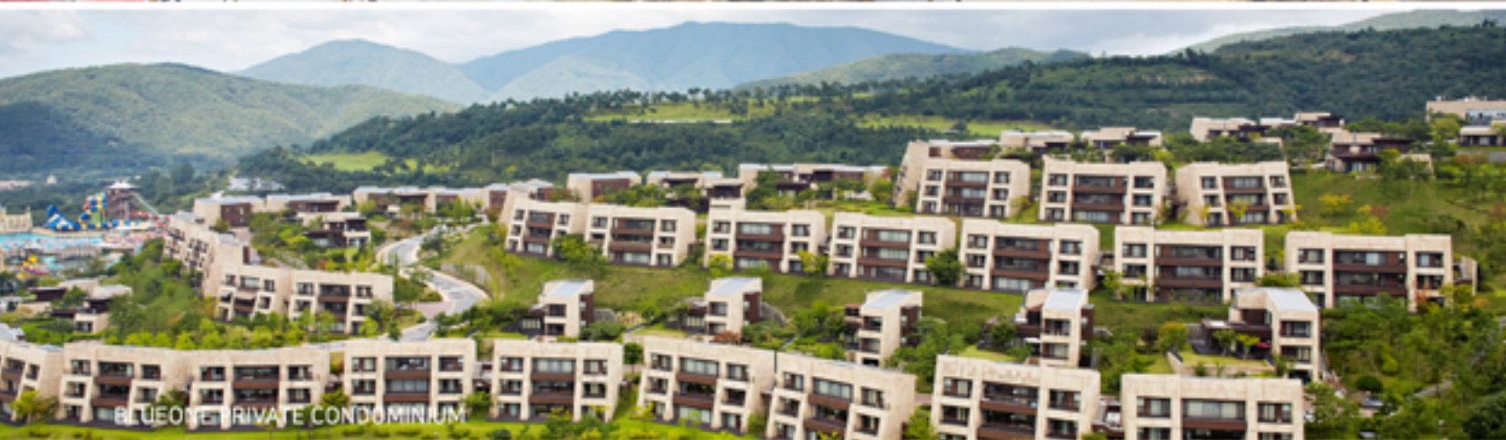
BLUEONE FAMILY CONDOMINIUM & WATER PARK
